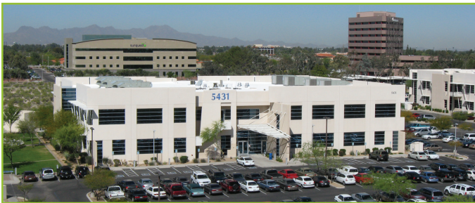
Aetna leased 12,239 square feet at 5431 E. Williams Blvd
